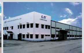
Hanoi factory (Vietnam) MV/LV switchgear, Mold TR
