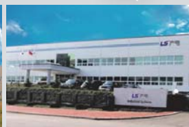
Dalian factory (China) MV/LV switchgear, MV contactor
