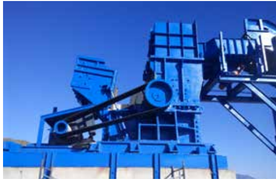
Jaw crushers Recovering and process plant Location: La Rioja, (Spain)
