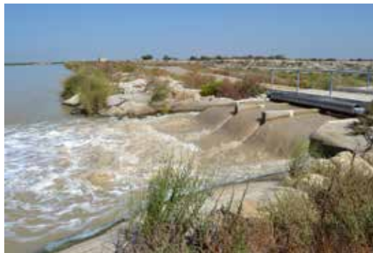
Trebujena solar pumping plant Location: Trebujena (Spain) Capacity: 1000 l/s
