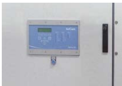
Lockable door prevents unauthorised access.
