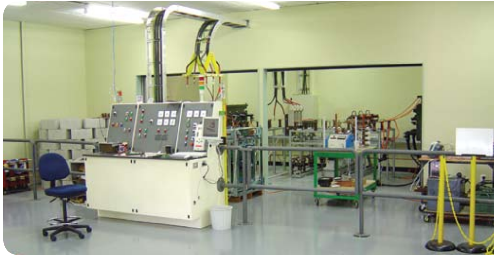
AuCom's medium voltage testing facility
