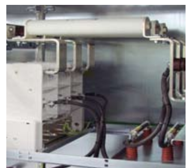
Contactors and fuse detail.
