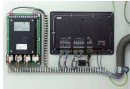
Fibre-optic cables isolate medium voltage and low voltage sections of the MVS and ensure 100% safety for operating personnel.
